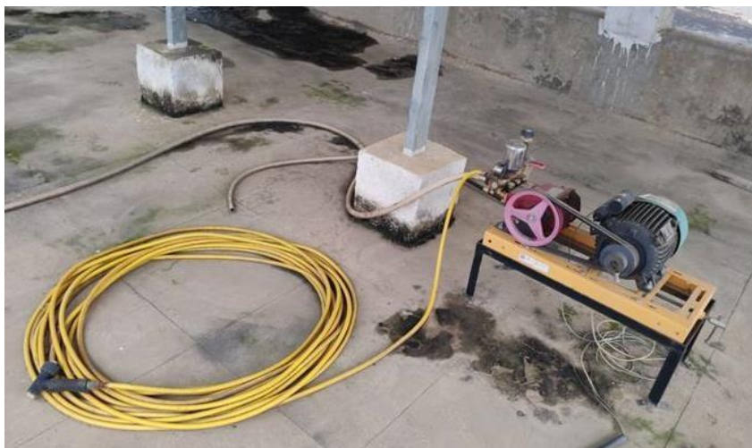
Figure 5-10 Pressurized water cleaning for SRTPV systems
