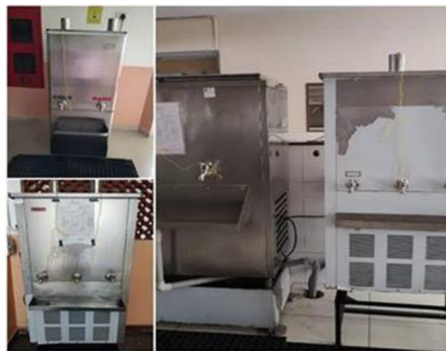
Figure 4-6: RO water treatment plant in the campus
