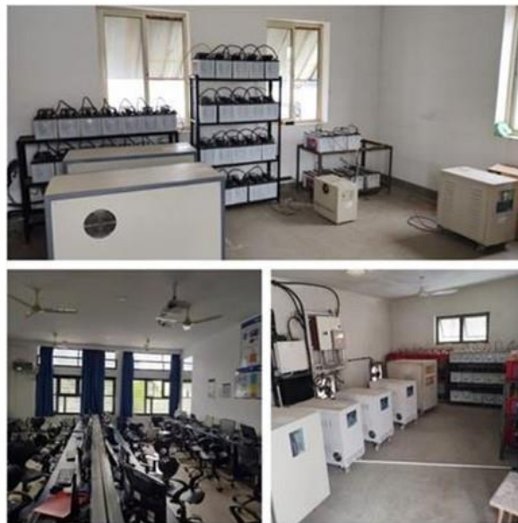
Figure 5-11: Well-ventilated and day-light integrated rooms
